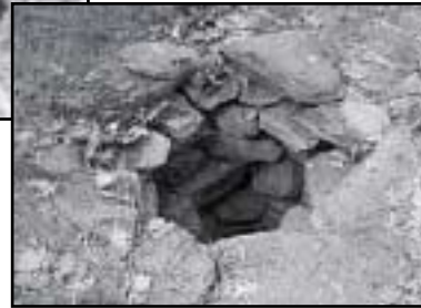
Unused and unmaintained wells threaten groundwater.
