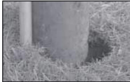
Faulty annular seal.
